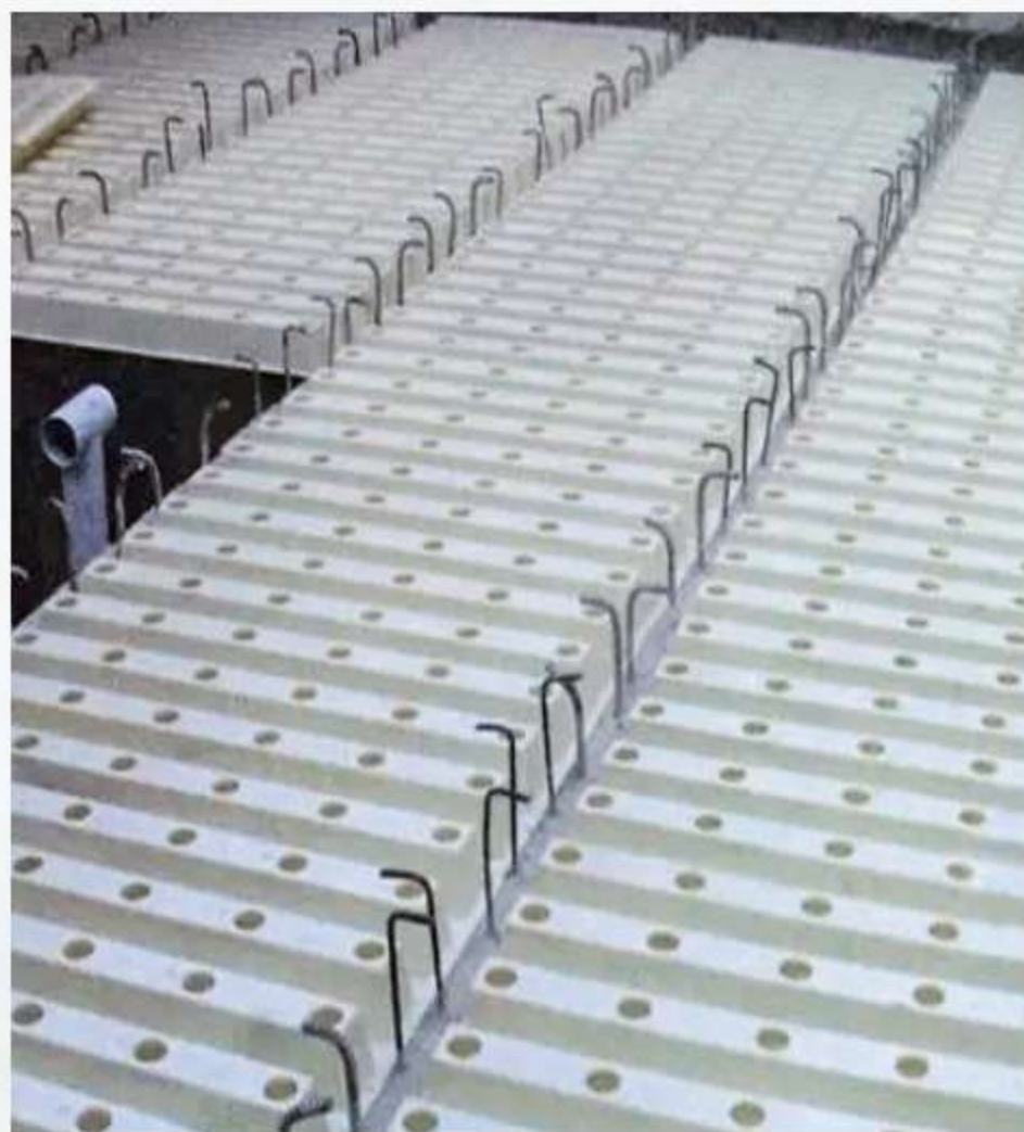
Integrally cast filter plate
