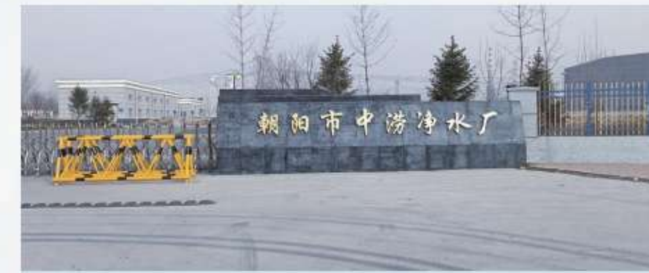
Chaoyang Zhonglao Water Treatment Plant Treatment Capacity: 100,000 m 3 /d Main Process: Coagulation + Sedimentation + Filtration + Disinfection
