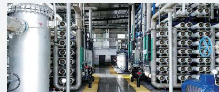
Yantai Economic and Technological Development Zone Water Supply Co., Ltd., Woniushan Water Plant Treatment Capacity: 67,000 m 3 /d Main Process: Ultrafiltration + Reverse Osmosis Dual Membrane
