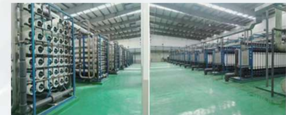
Ningdong Base Nanhu Water Plant Treatment Capacity: 38,400 m 3 /d Main Process: Ozone Oxidation + Chemical Softening and Sedimentation + V-Type Filter + Ultrafiltration + Reverse Osmosis
